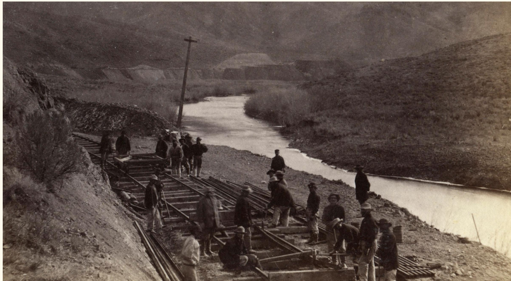
Laborers lay track along the Ten Mile Canyon stretch of the Transcontinental Railroad. Retrieved from Stanford University Libraries.
